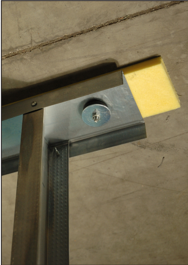
Isolate Top or Bottom of Stud Wall with Wallmat and Anchor Isolator (KAI)
