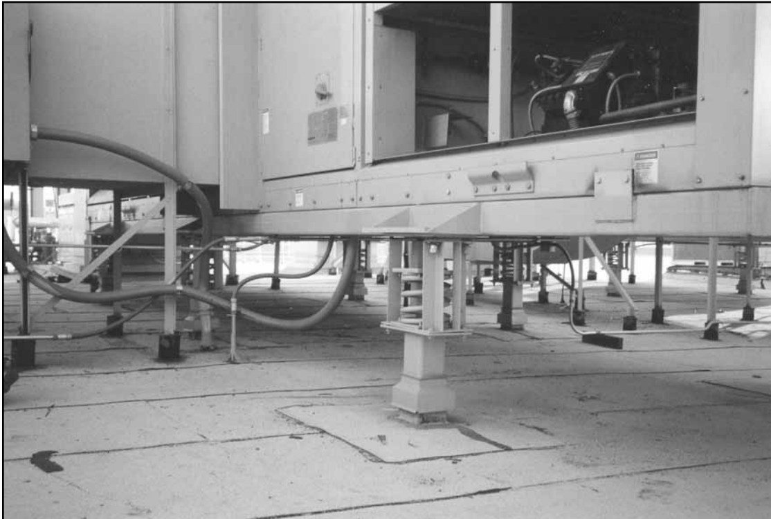
Kinetics FLSS rooftop isolation on a building in Culver City within one mile of the I-10 collapse.
