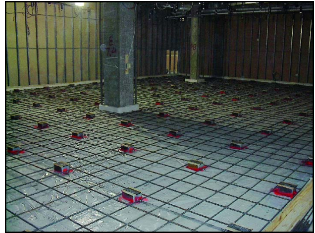
LSM Mounts and rebar; ready for concrete pour.
