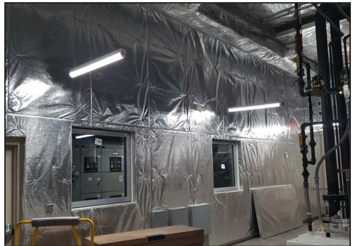
S4 Wall and Ceiling Installation in Generator Room
