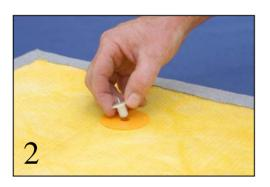
Insert marking plugs into the Snap-On anchors.
