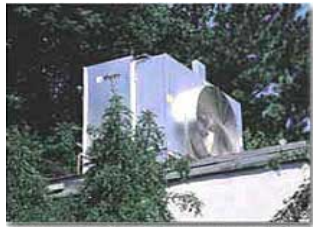
Figure 35: Fluid cooler cross flow with self-contained sump.
