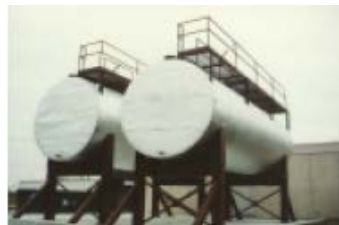
Figure 59: Horizontal tanks including concrete-lined tanks.
