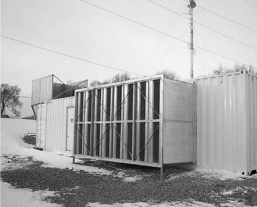
*Retrofit project using Model VRS rectangular intake silencers and Model STL barrier discharge silencing tunnel. The packager originally used a shipping container as the enclosure, with acoustical louvers. Due to the close proximity of residential land, increased noise attenuation was required.*
