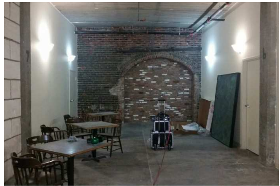
(Second floor lobby space used for original conditions testing)
